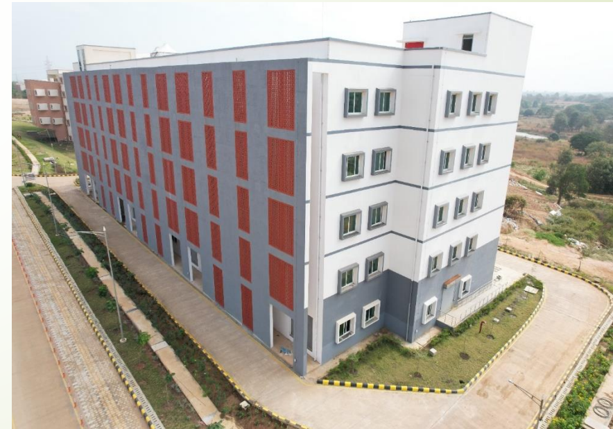
Central Instrumentation Facility (CIF)
